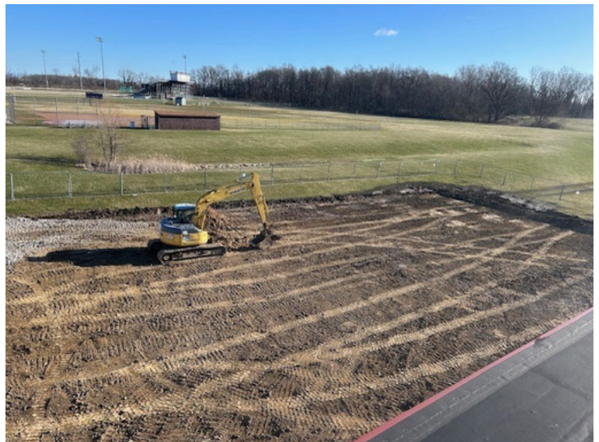
More construction photos
